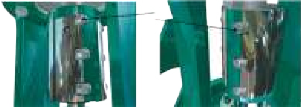
Figure 6.28 Placing and tightening the coupling screws.
